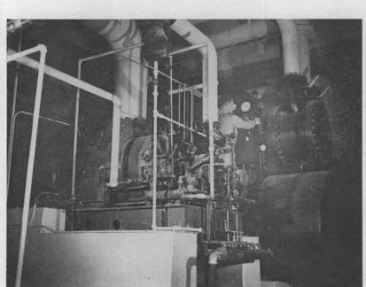
THE RIGHT TEMPERATURE for the entire building is maintained by the refrigeration air conditioning turbine. Here Harrel Killedrew, 2411, refrigeration mechanic, is shown examining the pressure gauges on the complicated mass of machinery.
